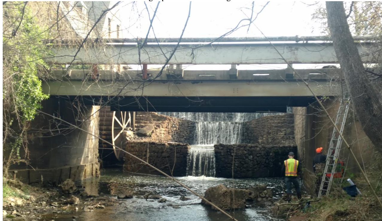
View Looking Upstream from Bridge No. 95
