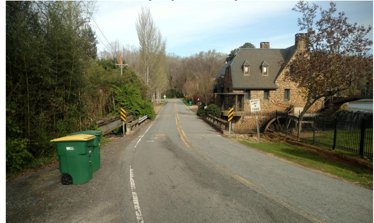
View of Existing Bridge No. 95 Looking Downstation
