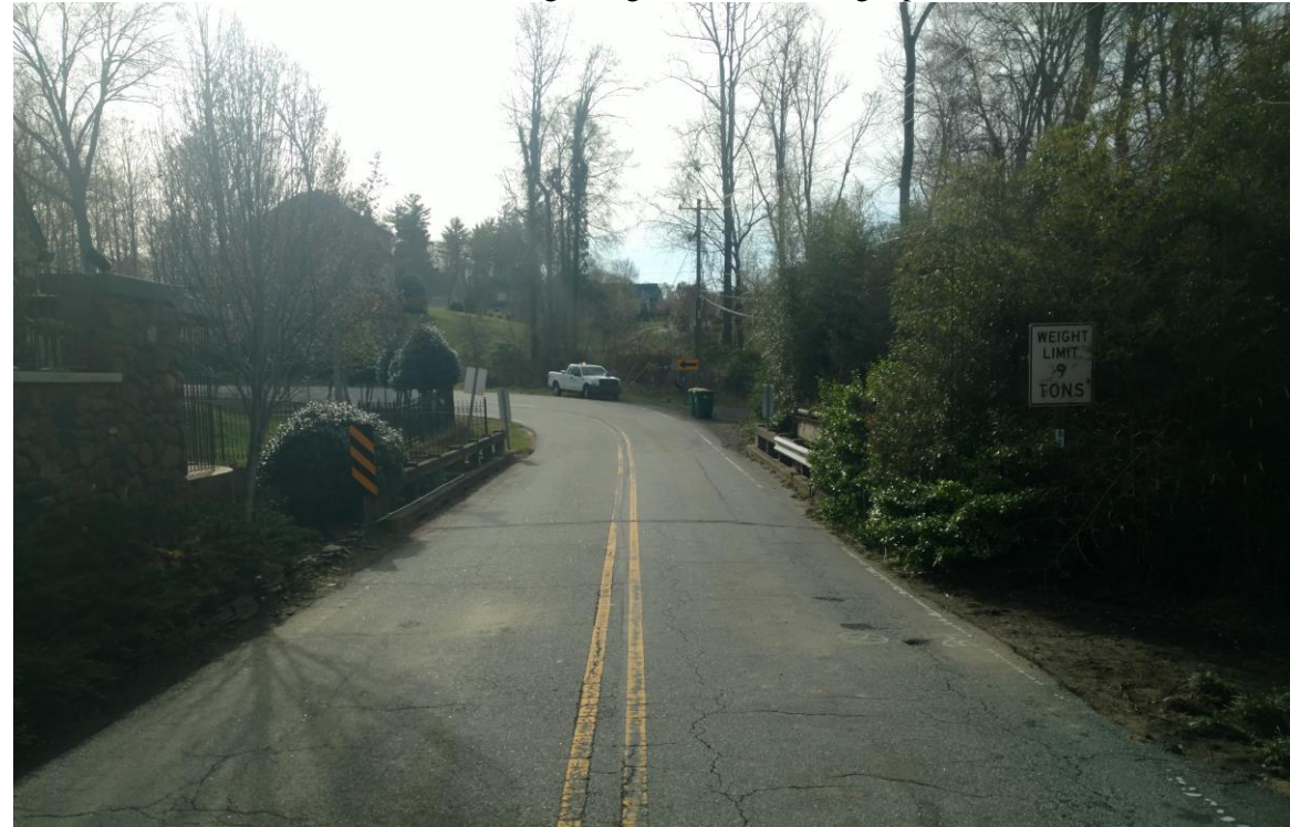
View of Existing Bridge No. 95 Looking Upstation
