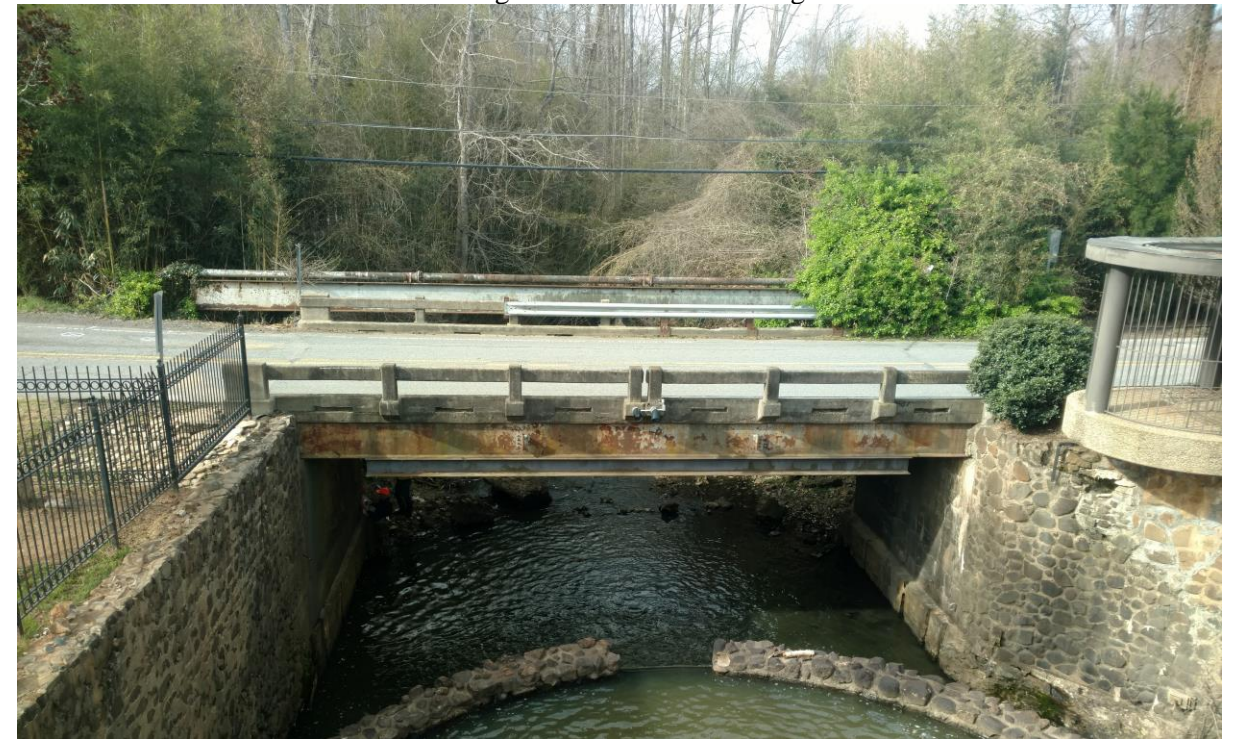
View Looking Downstream from Bridge No. 95
